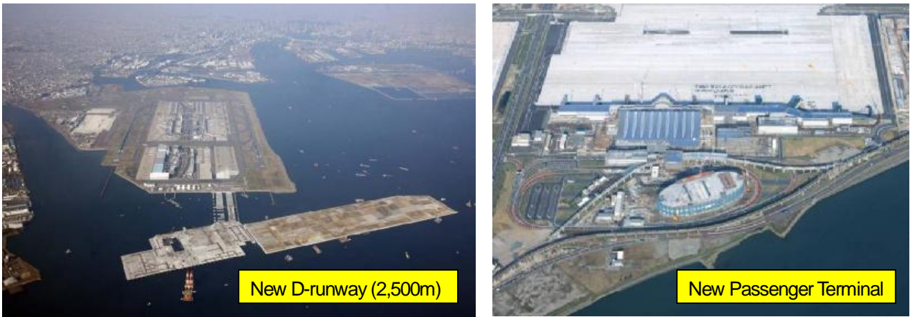
Figure 4: The construction of D-runway (left) and International Passenger Terminal Building (right)
